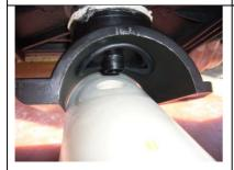
The air socket (19mm) of the upper clamp saddle part is inserted into the existing bore (25mm) of the pipe from above.
