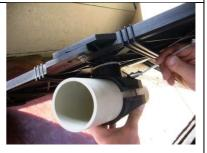
Now the clamp saddle is to be tightened by screwing (6 Nm) using a ratchet wrench.
