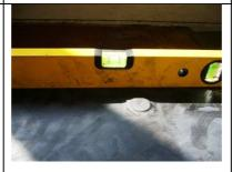
The diffuser has to be adjusted horizontally before the clamp is finally tightened.
