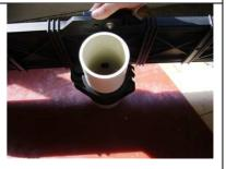
The clamp saddle has to be closed around the pipe.
